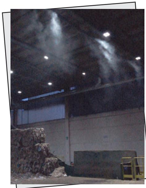
Misting systems are installed in painting units, quarries, mines, stone crushers, gravity flow places to conveying belts, truck yard ramps, hoppers unloading, suppression of dust produced by steel mills and cement factories, ships loading and unloading points, ores, rocks and coal storages, recycling plants and inert processing. Units will be placed near materials gravity drop places, where the concentration of fugitive dust particles is larger in diffusion and in surface.
