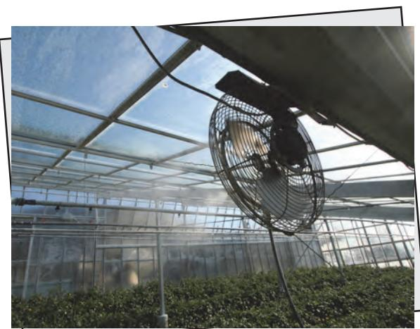
TecnoCooling fog system works on a pressure of 1000 PSI (70 Bar) and it is designed to produce water droplets smaller than 5-10 microns diameter that, for theirs dwarfish size remains suspended in the air for a long time producing the fog effect.
