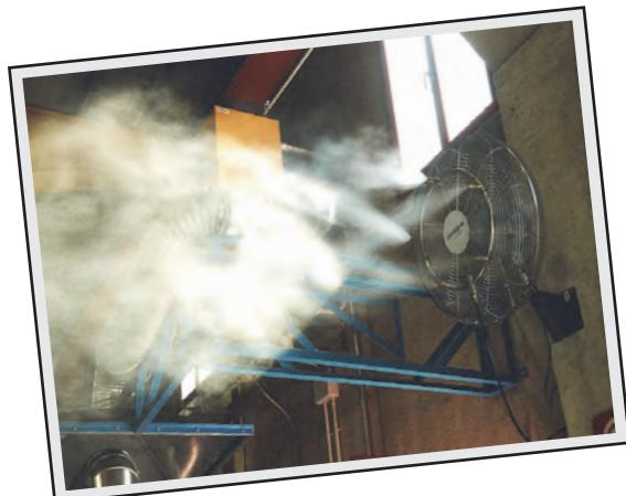
**Misting fans are the best solution for open areas, to provide air flow and cooling with the best efficiency. The two integrated systems, ventilation and misting, together ensure the best result against the high levels of relative humidity in the hot seasons.**
